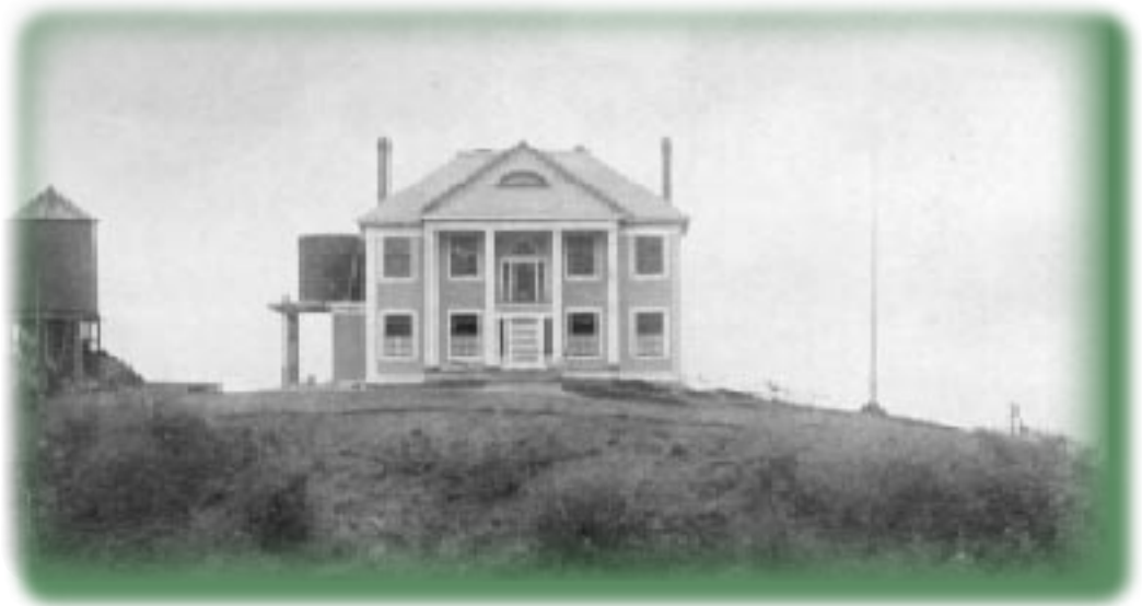
Sitka Station Building, 1902.
